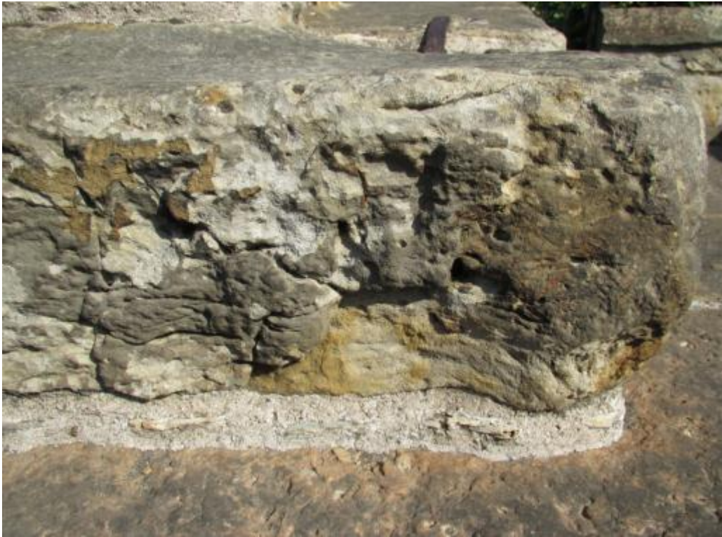
South side of upper step showing friable area
